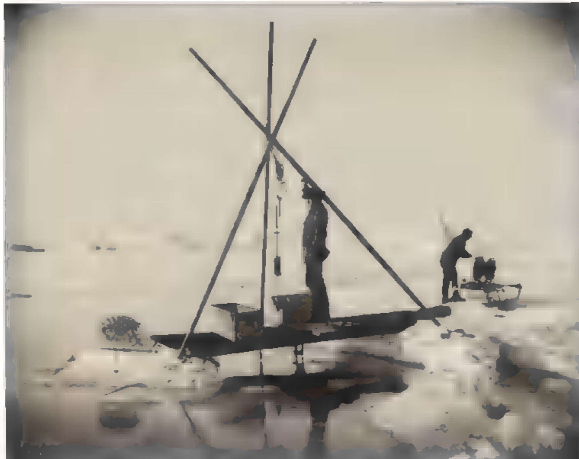
July 12, 1894: Nansen takes a reading of deep Arctic Ocean water temperature as part of the expedition's scientific work. Astronomical, meteorological, and oceanographic data were consistently collected.
